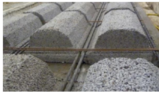
Figure 3. Close-up of block stones and reinforcement before casting strong concrete.
