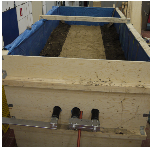
Figure 4.10: Experimental setup under construction. Three 245 kV XLPE cables with conductor cross sections of 1600 \text{ mm}^2 and lead screens are installed in an envelope of sand and surrounded by soil. In order to complete the setup, a layer of soil was installed on top.
