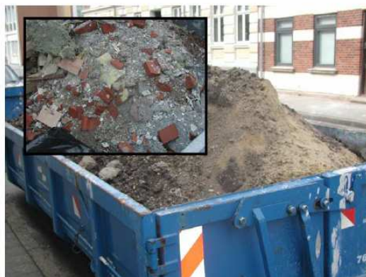
Fig. 14. Construction materials meant for recycling, but partly contaminated by PAH from earlier tar impregnation. Insert shows an example of this most difficult lot heterogeneity manifestation. Even such “impossible-to-sample” problems are doable in the context of TOS however, see text.
