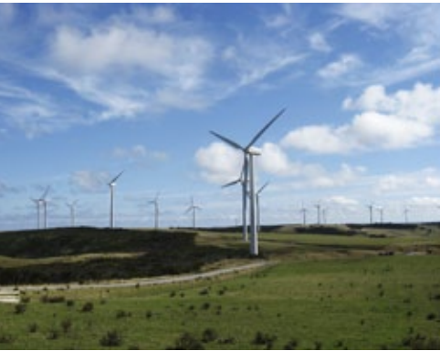
WoolNorth Wind Farm, Tasmania 19
