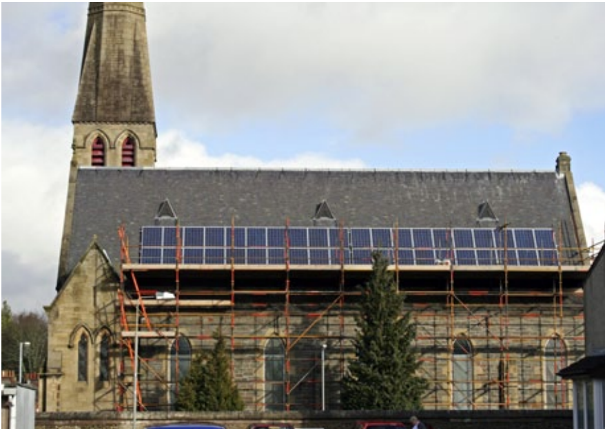
Solar panel installation on a church roof 38
