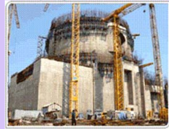
2X1000MWe VVER reactors under construction at Koodankulam (Going Critical in 2008)
