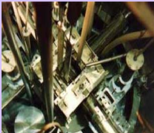
Inside view of Kamini reactor, 100 MW Went critical in Sept 96, using U-233 fuel
