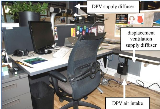
Fig. 1 DPV installed at one of the workstations
