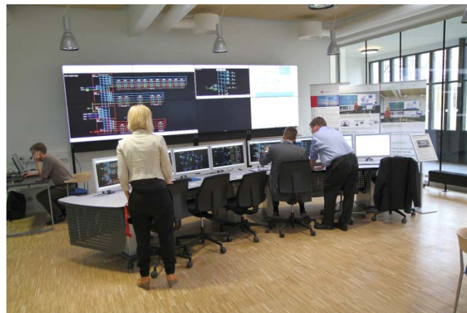
Figure 4. ControlLab + Scada system for education and research. The Scada system allows for monitoring and control of the main laboratory facilities including monitoring of the electrical power system on the island of Bornholm.
