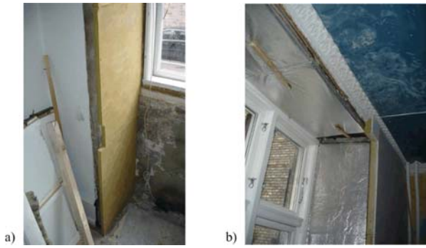
Fig. 7. Insulation applied in the window reveals where a) is Aerowolle and b) is Vacupor NT
