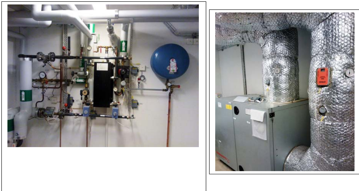
Figure 5. District heat plate heat exchanger sub-station installed at building ground level (left), and installation for exhaust air heat recovery to inlet air (right). Photos: The Author.
