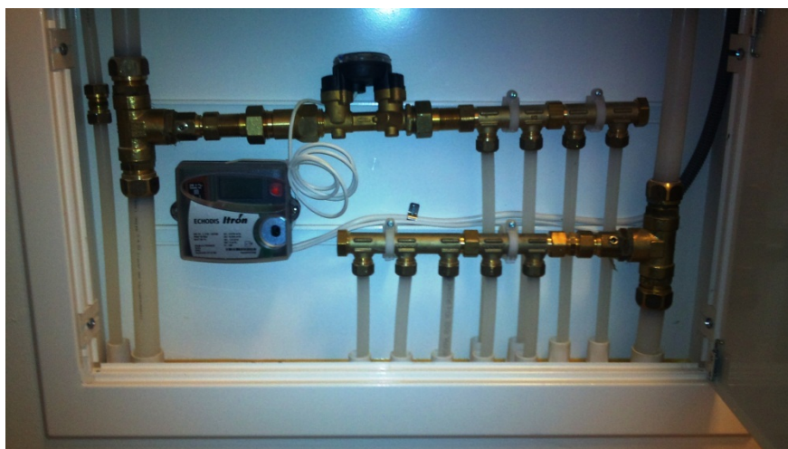
Figure 8. Installed equipment to facilitate individual metering of DHW use in each apartment. Photo: The Author.
