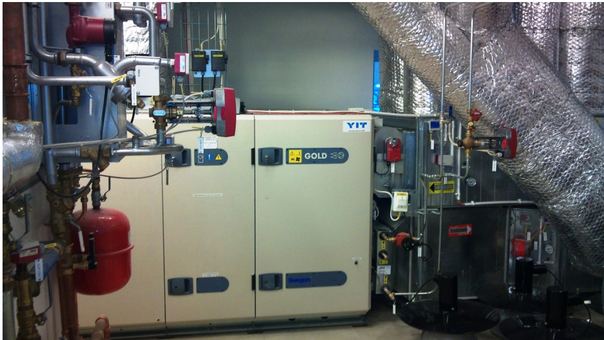
Figure 6. Forced air ventilation system with centrally placed rotating heat exchanger and subsequent district heat added as base load heat supply. Photo: The Author.
