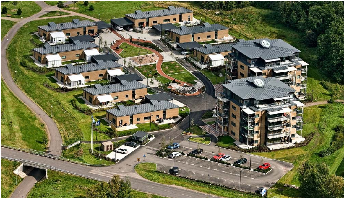
Figure 11. The Söndrums Kyrkby multi-family and pair passive house settlement in operation. Source: [11].
