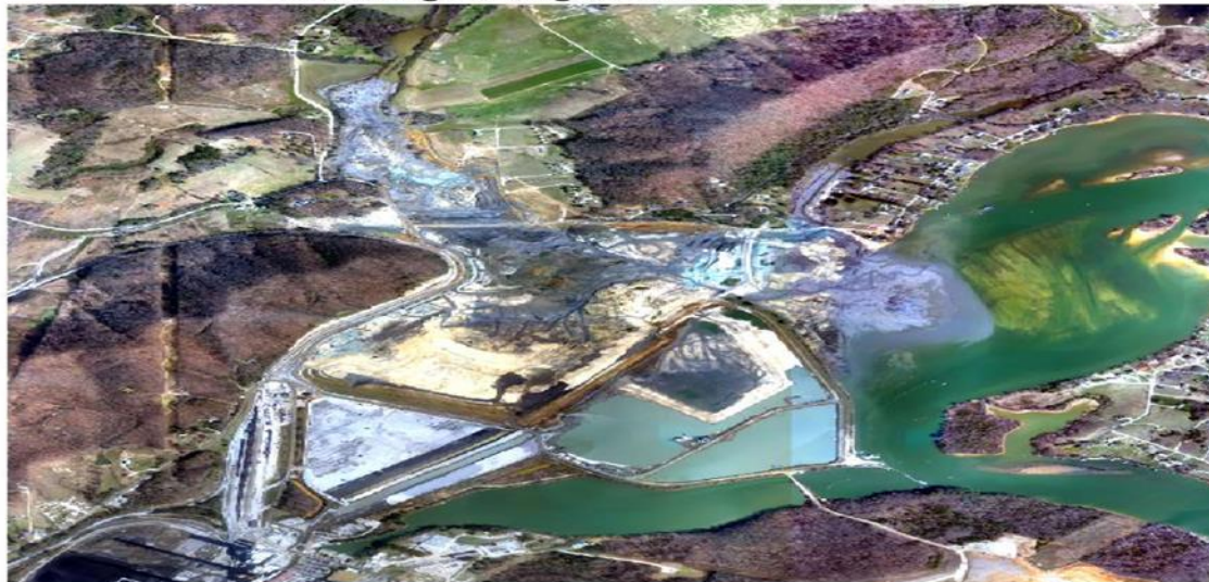
Aerial Image of Kingston Ash Slide 03/20/2009
