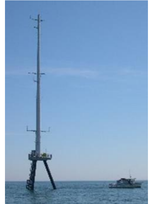
179 feet installed at Horseshoe Shoal
