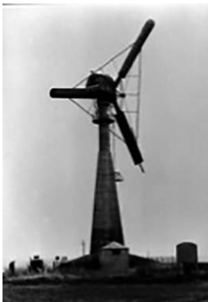
Figure 3. The Gedser wind turbine (© Elmuseet, Bjerringbro)
