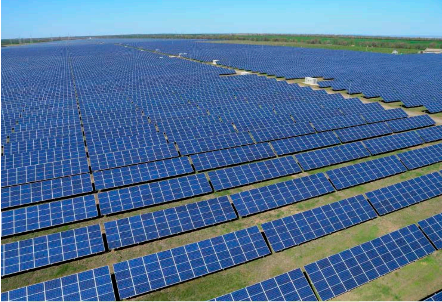
Photo credit: Activ Solar
