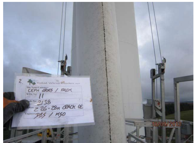
Figure 3 Front edge cracks (transverse and longitudinal)
