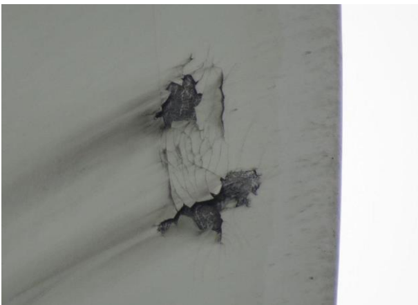
Figure 8 Missing external parts
