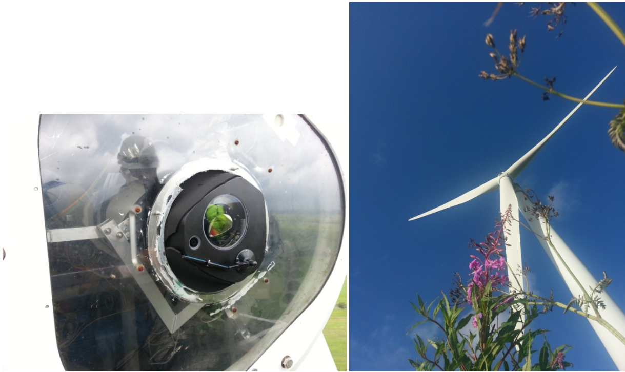
Figure 11. Left: SpinnerLidar during installation in Dong Energy's NM80 Test Turbine at Tjæreborg Enge (July 2012) Right: NM80 2.3 MW Test Turbine at Tjæreborg Enge, Jutland, Denmark owned by Dong Energy.
