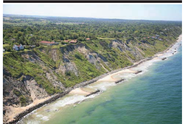
Figure 2. NE Sealand coastline with older as well as new houses on the cliff top (Photo: DCA/Hunderup Aerial Photo).
