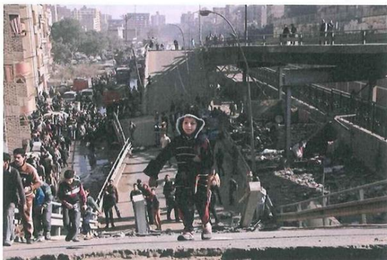
People stand on a collapsed bridge in Cairo on Tuesday. Political turmoil has led to a deterioration of infrastructure. El Shorouk/Associated Press
