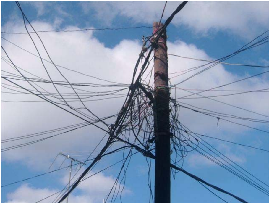
In most slums, electricity is accessed through informal connections. These are often precarious and home-made solutions, presenting many health risks which the private distribution companies do not take legal responsibility for.
