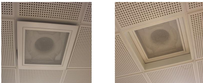
Fig. 2 Fan coil position in baseline condition (left) and in diffuse ventilation condition (right)
