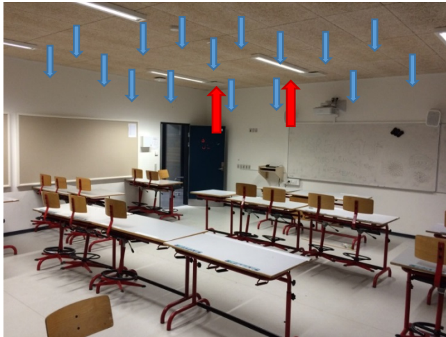
Fig. 2 Photo of classroom #1 with a diffuse ventilation ceiling. Three exhaust grilles are placed in the ceiling in a line parallel to and above the white board. Only two of exhaust are visible on the photo.
