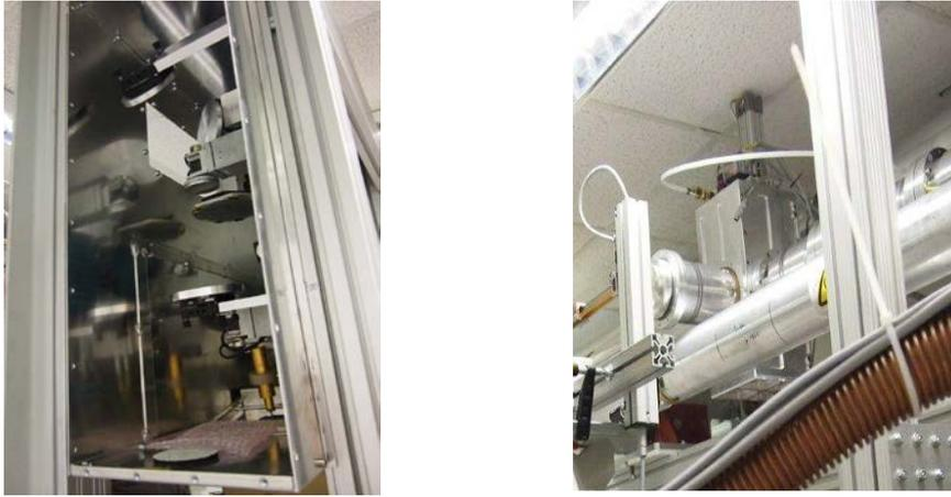
Figure 20. Photographs of the installed receiver box (left) and the RF switch installed in transmission line (right).
