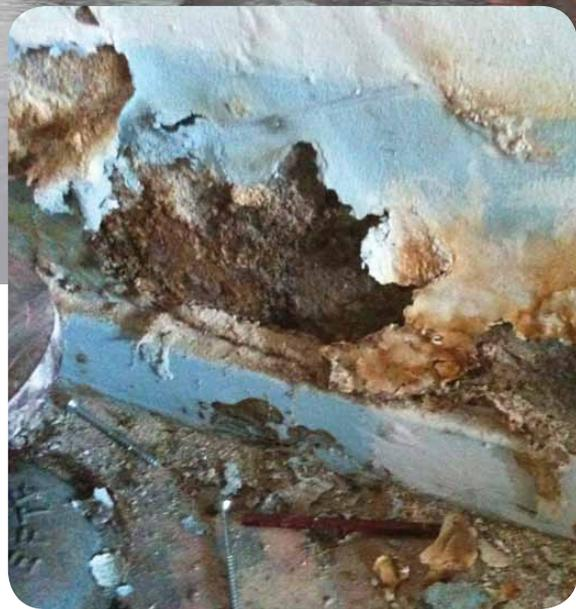
Typical damage due to water penetration through basement walls. Photo: Rimante Andrusiunaite Cox.
