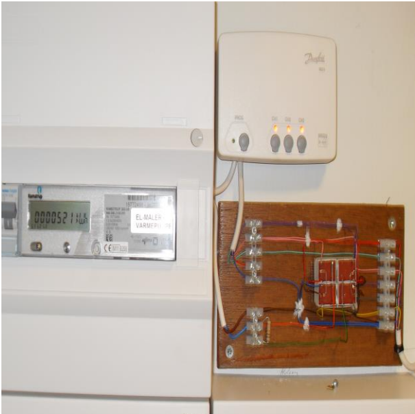
Figure 1. Jens observed that DE often only optimised his heat pump once a day, so he made an electric hob that allowed him to optimise twice a day.
