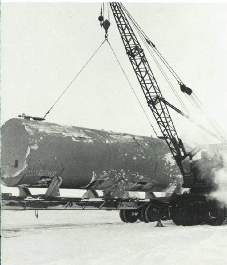
Fuel tank being lifted onto flatbed by crane.
