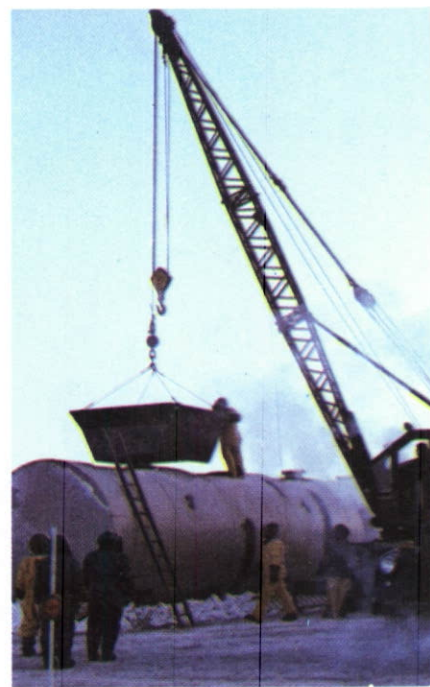
Crane lowering a chute onto 25,000-gallon tank preparatory to loading it with contaminated snow and ice.
