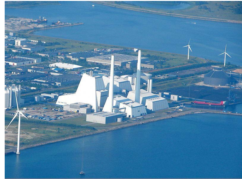
Avedøreværket, a combined heat and power plant
