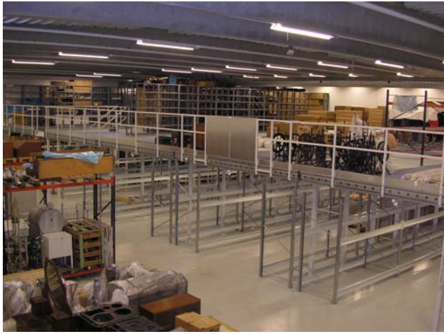
Figure 6. Picture of the interior of the museum storage showing the mezzanine construction (Photo Centre for Preservation of Cultural Heritage).
