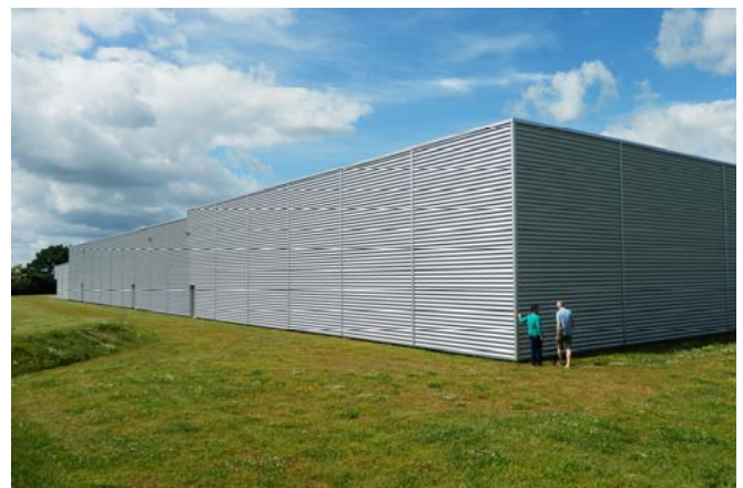
Figure 8. Exterior view on the storage building after completion. Old to the left and New to the right (Photo Christensen).
