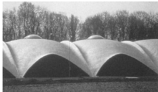
Figure 4. Tennis halls designed by Heinz Isler.
