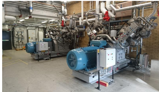
SPP HighLift heatpumps installed at AstaZeneca in Mölndal, Sweden
