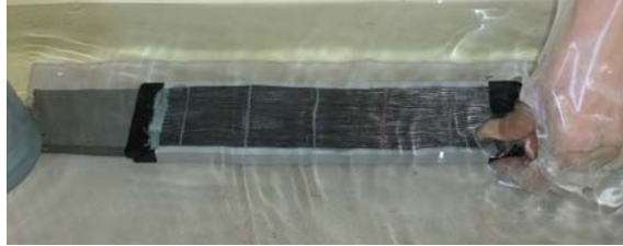
(b) CFRP strand sheet placement
