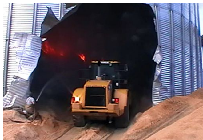
Top: Water is often an unsuccessful method of fighting smouldering fires in bulk storage silos.
