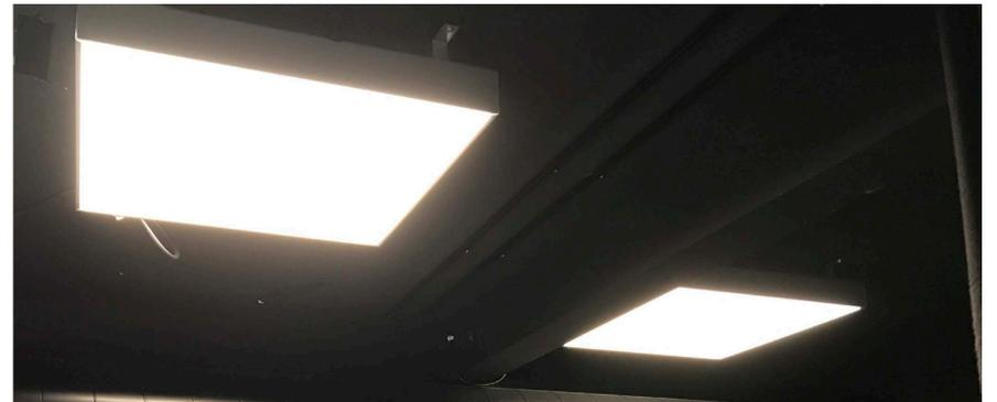
Figure 1 - Two 60x60 cm ceiling LED lamps in a facility at DTU used as an authentic example. The lamps are dimmable using pulse width modulation, however using slightly different frequencies. The left lamp (lamp 2) exhibit 551.8 Hz and the right lamp (lamp 1) exhibit 546.7 Hz.
