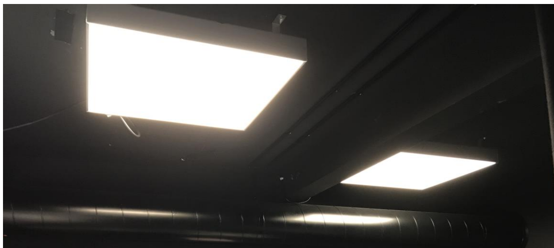
Figure 1 – Two ceiling lamps in a facility at DTU used as an authentic example. The lamps are dimmable using pulse width modulation, however using slightly different frequencies. The left lamp exhibit 551.8 Hz and the right lamp exhibit 546.7 Hz.
