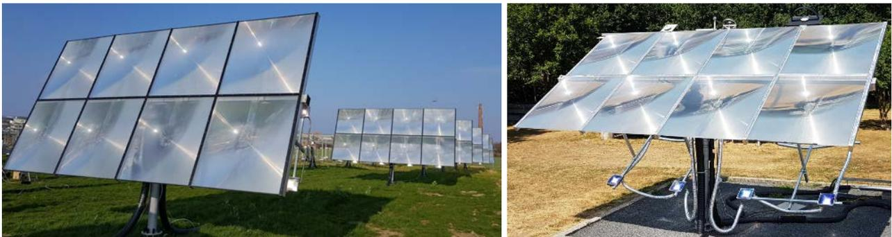
Figure 1c. Actual installation on Møn, Denmark (a 2 MW solar field for district heating purposes) and at DTU Civil Engineering's test facilities in Kongens Lyngby, Denmark.
