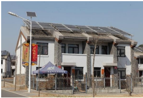
A farmhouse heated by solar energy
