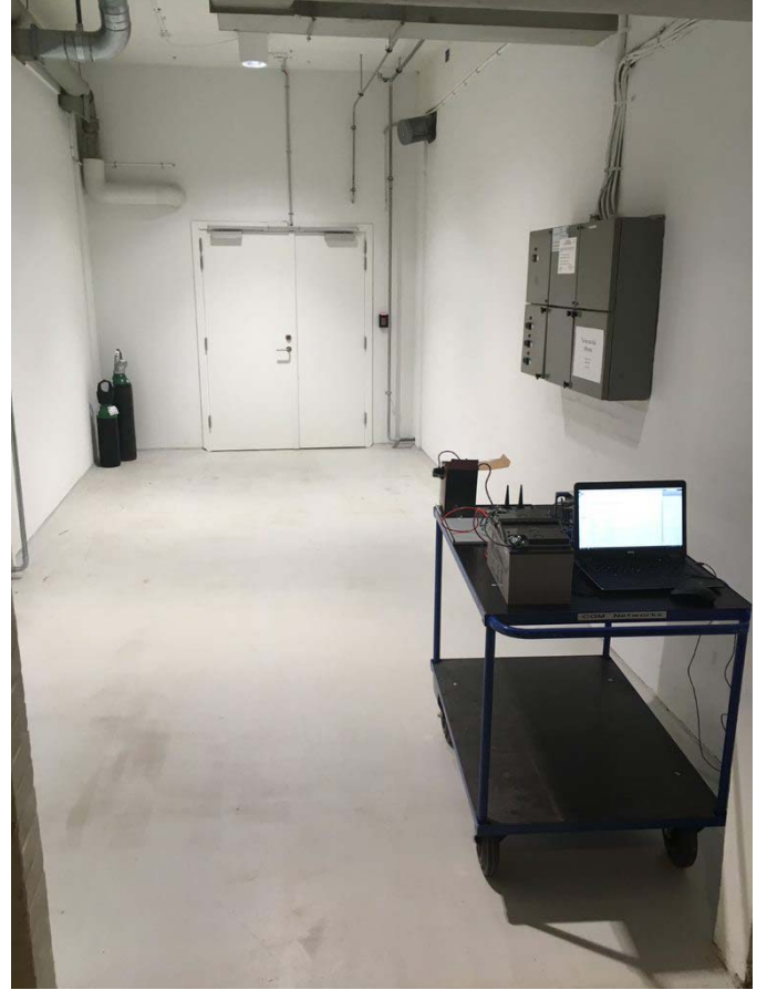
Fig. 5. Measurements in the basement of building 340
