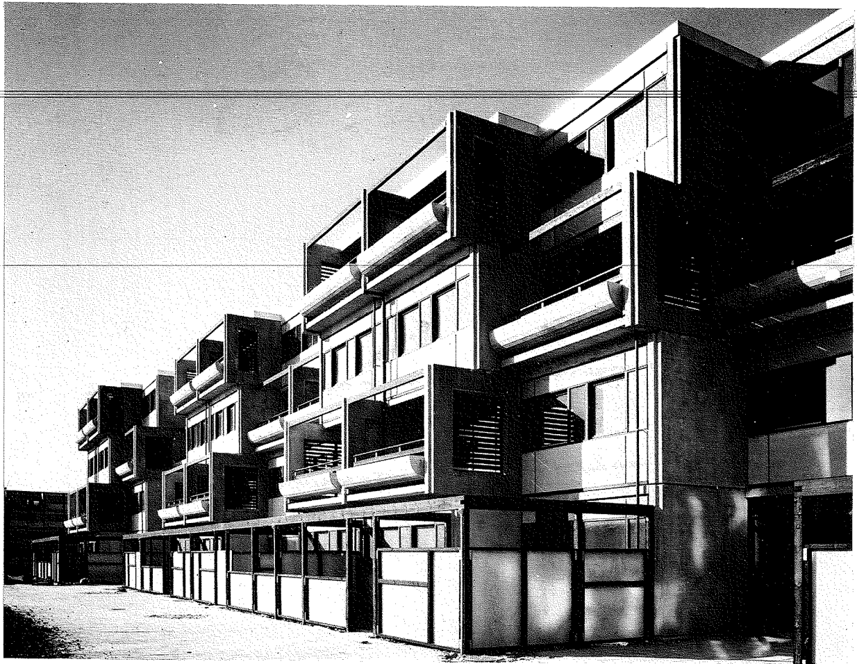
Figure 11. BRØNDBY STRAND. See text and figures 9-10. Svend Høgsbro, Architect, M.A.A., A/S Dominia, Larsen & Nielsen A/S.
