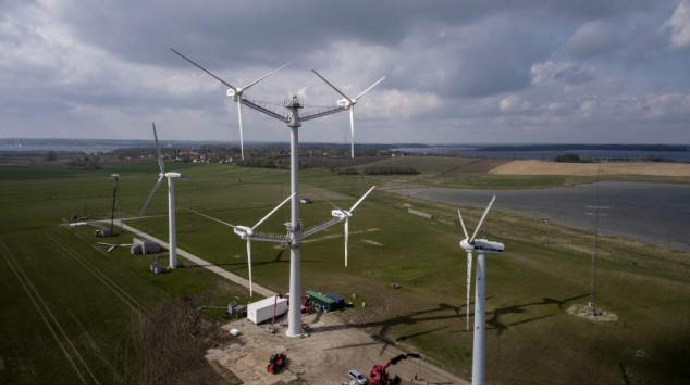
Fig. 1. Vestas MRT demonstrator, consisting of 4 V29 225 kW nacelles and rotors. Courtesy of Vestas Wind Systems A/S.
