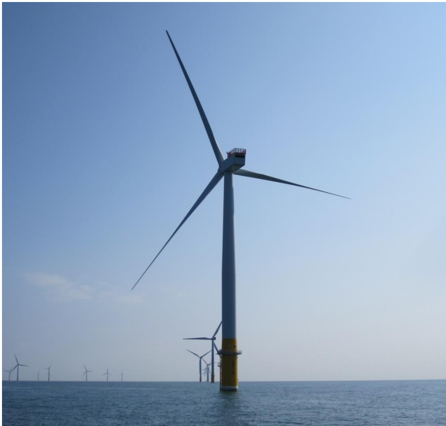
Figure 4 View from turbine IGF10: East
