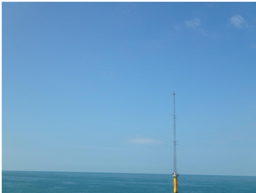
Figure 5 View from turbine IGF10: South – West
