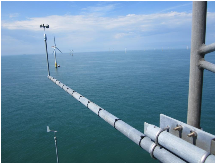
Figure 6 View from turbine IGF10: North – West
