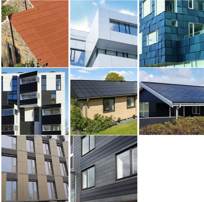
Figure 3. Examples of colored solar panels sold in Denmark. Top row (from left to right): CFR Energy panels, 11 Solaxess façade panels, 12 and Kromatix/SolarLab panels. 13,22 Middle row (from left to right): Racell panels, 14 Ennogie-taget panels, 23 and an xs-roof panel. 24 Bottom row (from left to right): Skala panels 15 and Zappa panels. 25
