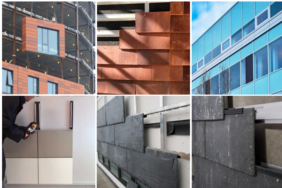
Figure 1. Top row: Existing mounting systems (from left to right): prefabricated façade system (CSR), 2 ventilated façade system (Komproment), 3 and curtain wall (HSHansen). 4 Bottom row (from left to right): Mounting methods for ventilated façade panels (from left to right): Sikatack panelsystem, 5 Komproment, 3 and Komproment. 3
