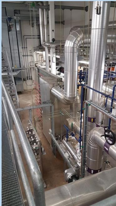
Fig 1. Future energy systems will rely as much on data as on the pipes. Heat exchanger for district heating in Tingbjerg (Copenhagen), one of the cases in the IDASC project.
