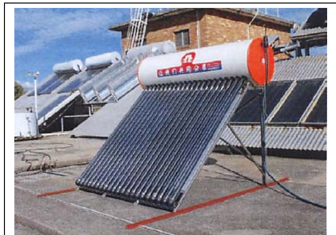
Figure 5. Water-in-glass solar water heater.
