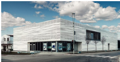
Heat pump system located in Maskinrummet, Århus Ø, Denmark [Kollision, 2020].
