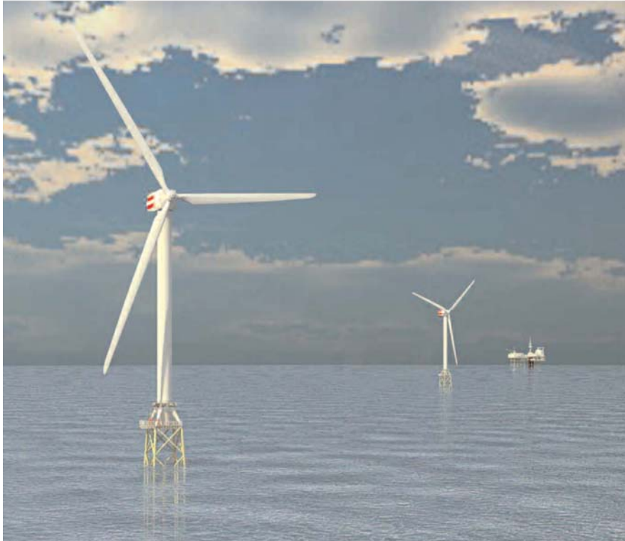
Figure 28: The Beatrice wind farm consisting of two 5 MW wind turbines in 42 m deep water. The wind farm is connected to an existing oil production facility. Source www.beatricewind.co.uk
