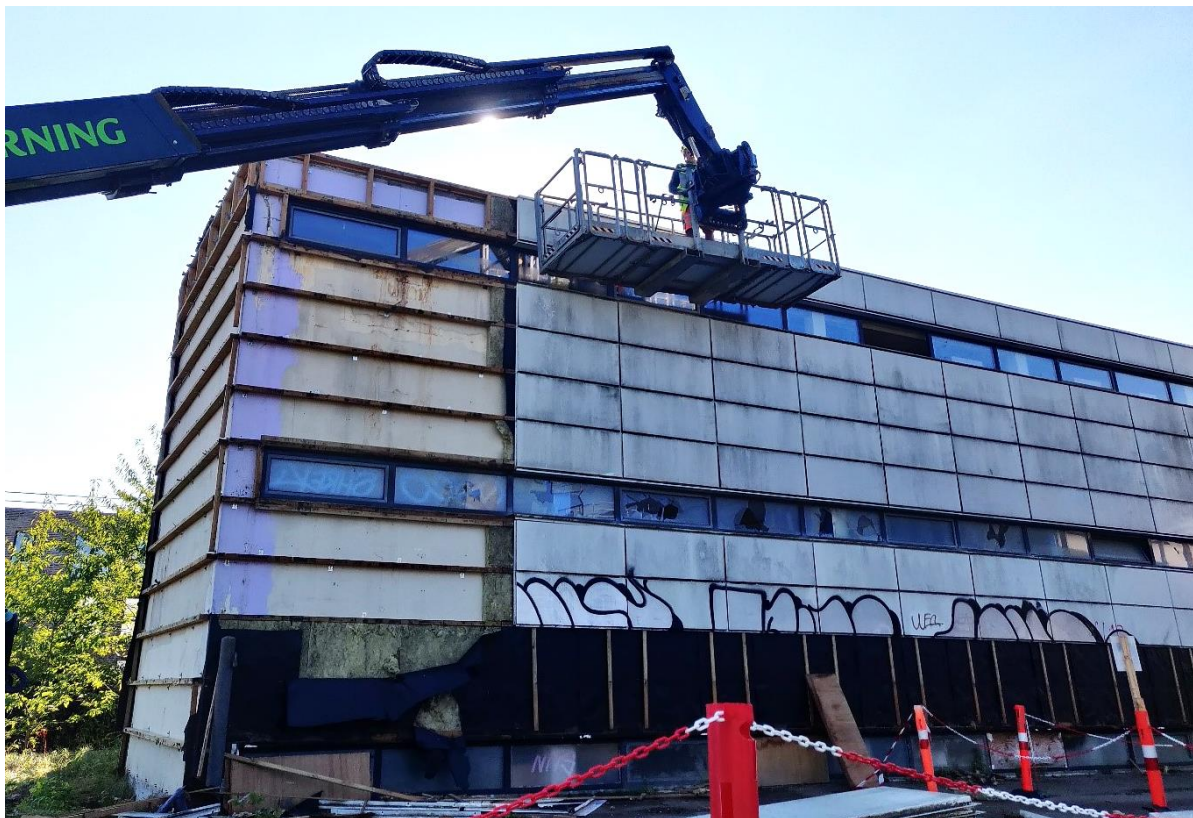
Figure 21. Selective demolition of façade cladding using a mechanical lift (Photo provided by Tim Riis Tolman, Lendager TCW).
