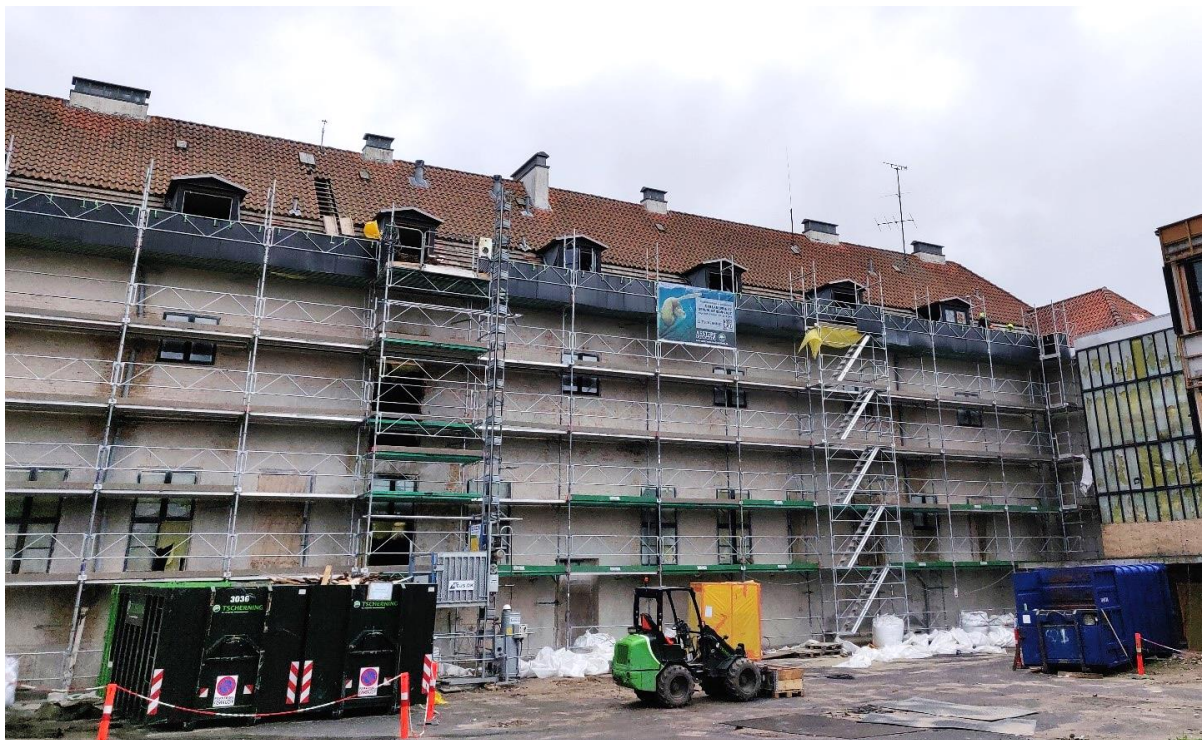
Figure 20. Selective demolition of roof tiles using scaffolding (photo provided by Tim Riis Tolman, Lendager TCW).
