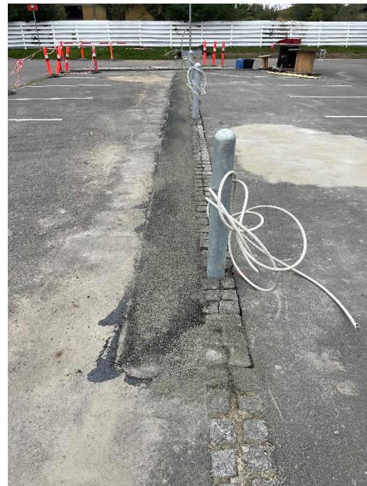
Figure 9: Poles are ready for installation of chargers.
