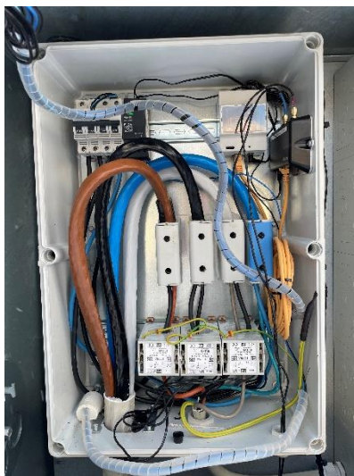
Figure 11: Cable cabinet installed at Campus Bornholm (top), and equipment inside the cabinet (bottom).
