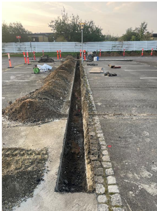
Figure 7: Preparing the parking lot for installation of cables.
