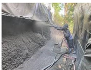
(a) Ground support walls
