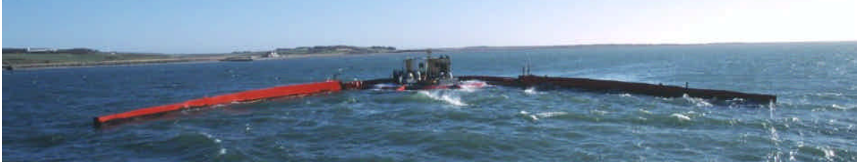
Figure 2: Wave Dragon prototype. Approaching waves are concentrated by the reflector towards the ramp
