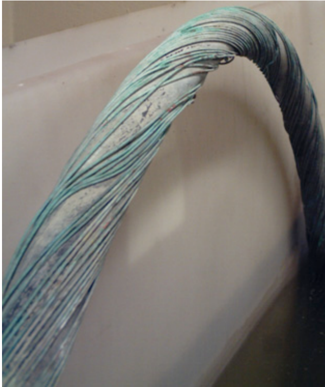
Fig. 1. Cable sample P3. Note the rather loose shield.
