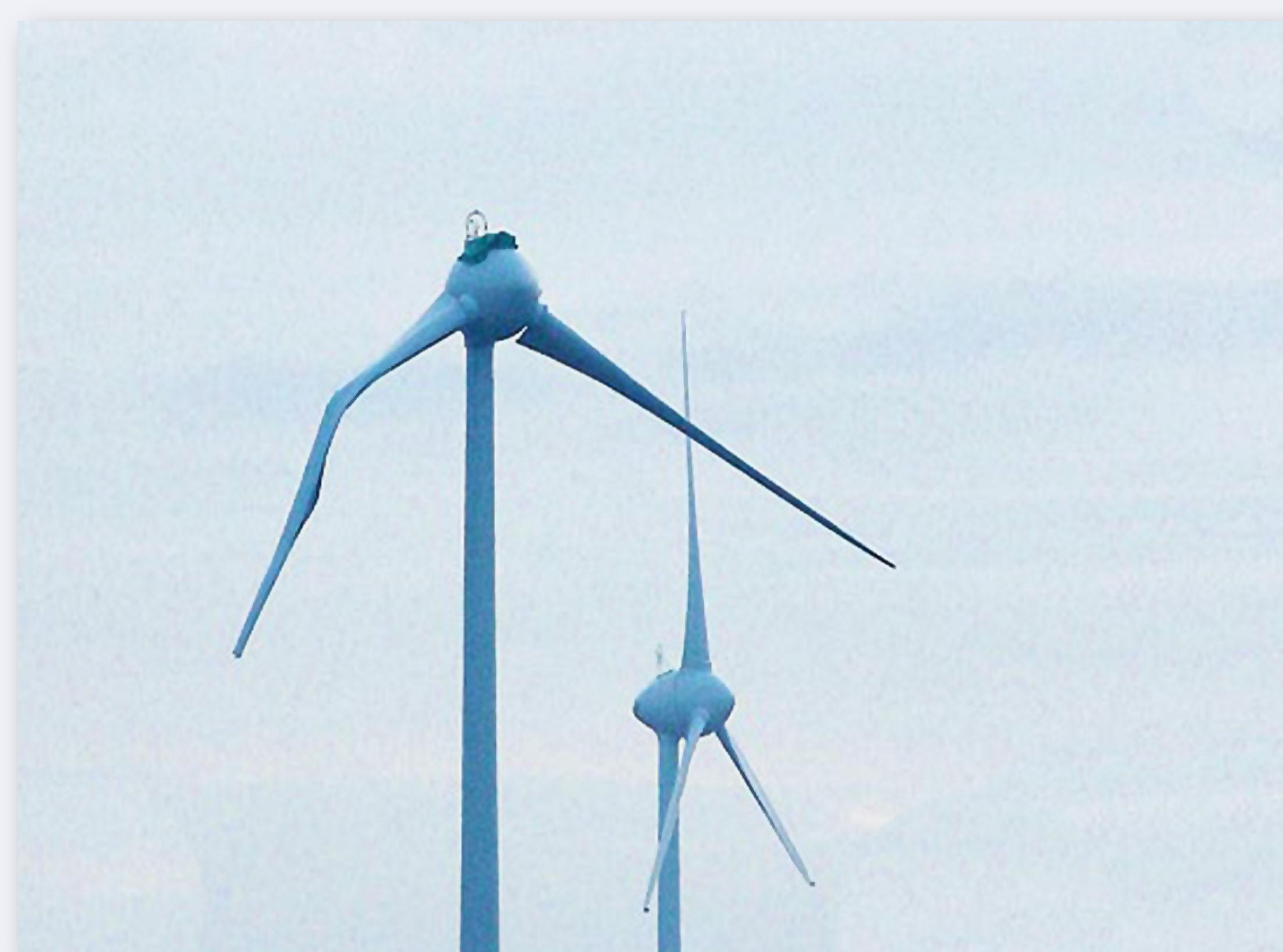
Figure 1: Broken wind turbine ( www.thesun.co.uk )
