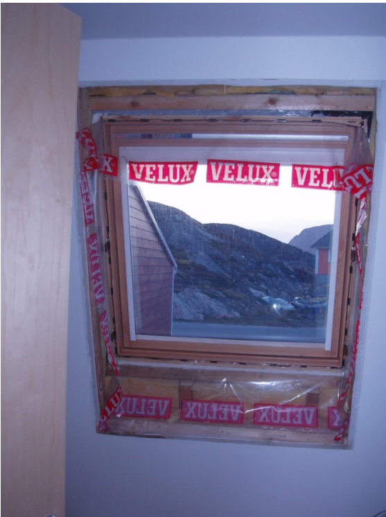
Figure 32 Fixing of skylight windows
