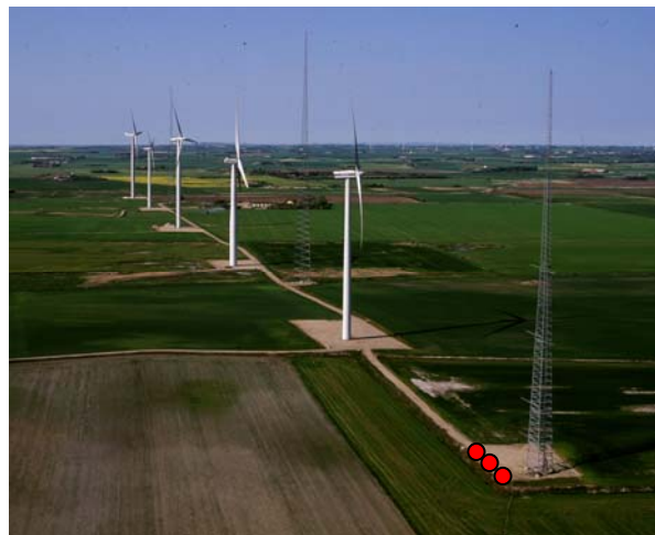
Figure 19 : The row of wind turbines at Høvsøre with the 116.5 m meteorological tower in the foreground. Lidars under test are placed along the road next to the metrology tower as indicated by red circles. The picture is taken from a low flying aircraft to the south-west of the mast. The five westerly masts dedicated for turbine studies cannot be seen in this picture.
