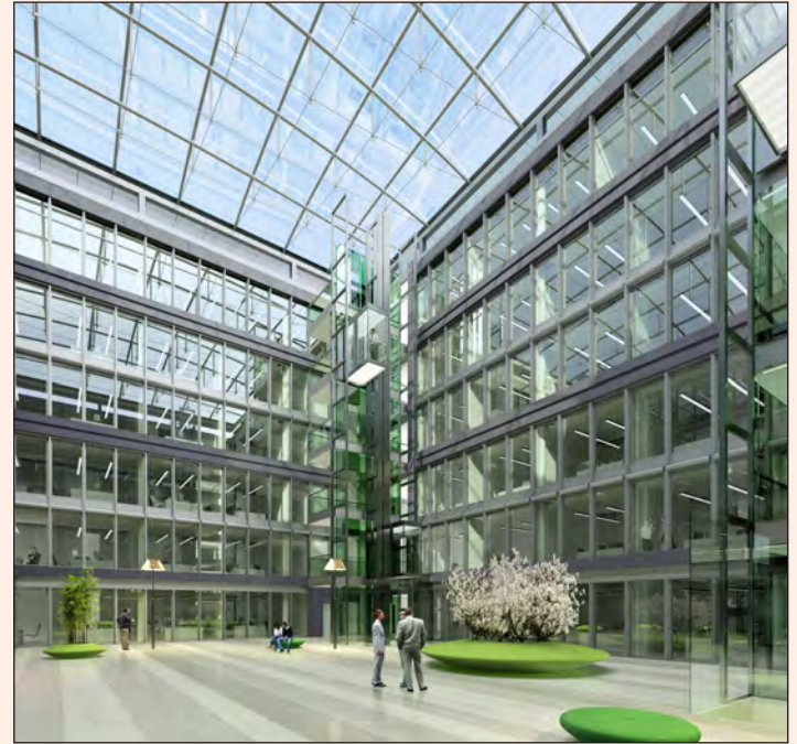
A view of the high, bright atrium. The atrium's underfloor heating and the heaters of the air conditioning systems are supplied via heat pumps.
