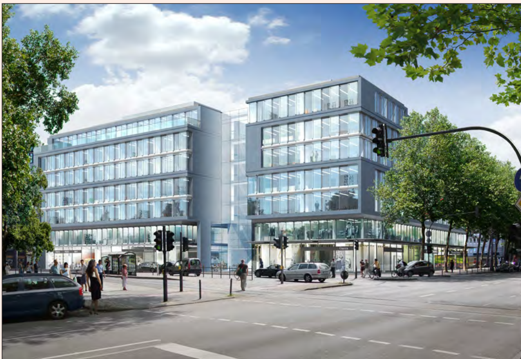
The Westgate in the center of Cologne has been certified by the European Commission as a 'Green Building' while still in the construction phase. It will consume 32% less primary energy and emit 53% less carbon dioxide than a comparable building.
